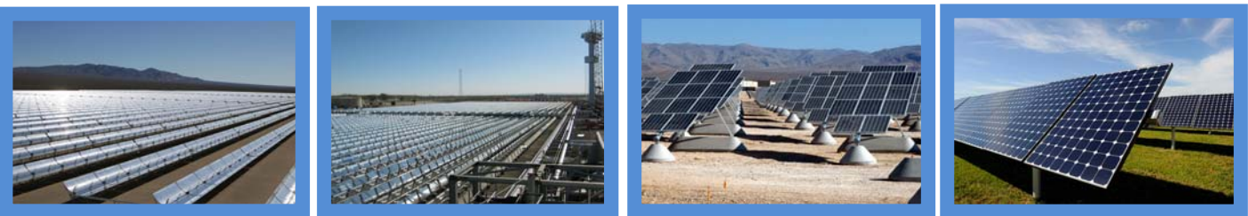
Nevada Solar One
